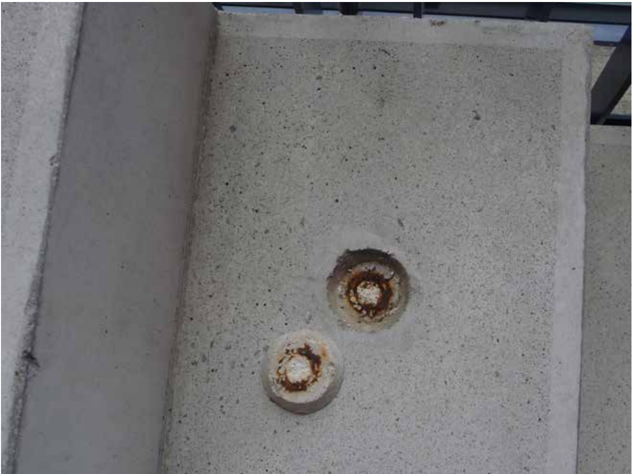
offene Transporthülsen Treppe
